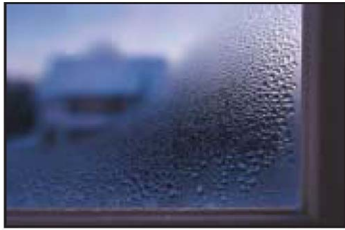
Condensation on the inside of a windowpane.
